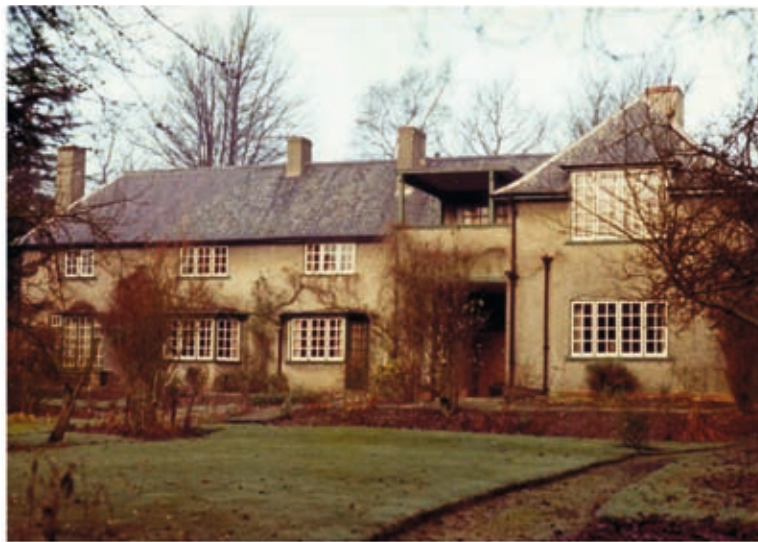
The Grey Cottage from the rear in 1972. It was demolished in 1981, but Sherrif Cottage next door, where Sir Granville Bantock lived, is still there.
